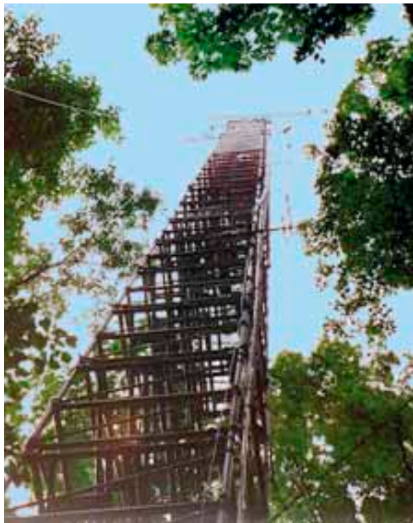
Figure 17. Eddy covariance tower in Manaus, Brazil, measuring fluxes of CO 2 , water vapour and energy.
