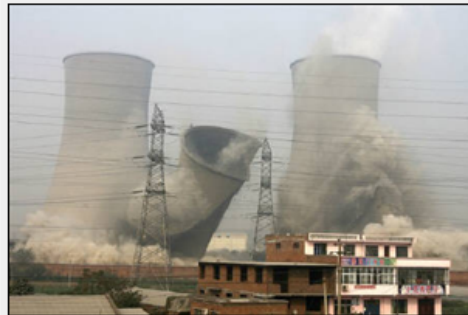
Cooling towers are demolished in an attempt to save energy and reduce emissions, at a power plant in Xinxiang, Henan province, October 28, 2009. REUTERS/Donald Chan/Files
