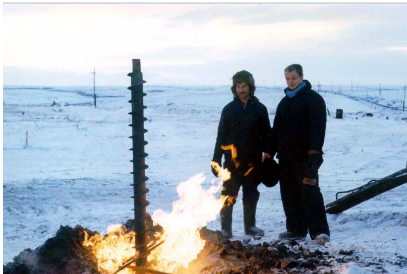
Fire when drilling monitoring well
